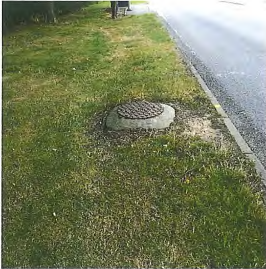
Beehive Lane, looking north east. Stats cover will need to be altered to match proposed finished surface level
